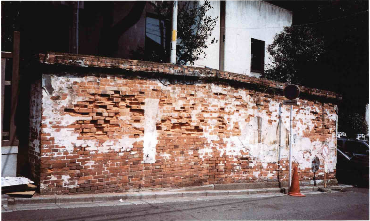
タフォニ状風化調査地の赤レンガ壁面 Red Brick Wall to Tafoni Weathering Studied in Tokyo, Japan Wide 8m18cm Left high 2m36cm Right 2m 61cm
